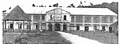
The Palácio site in 1900. The corrugated iron roof is in place.
