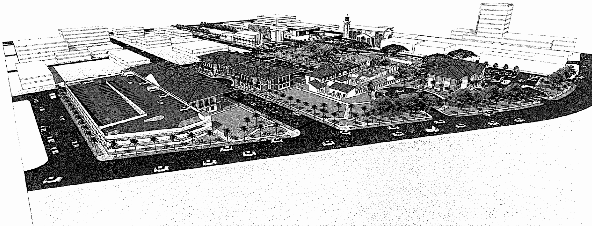
AERIAL VIEW FROM SOUTHWEST
