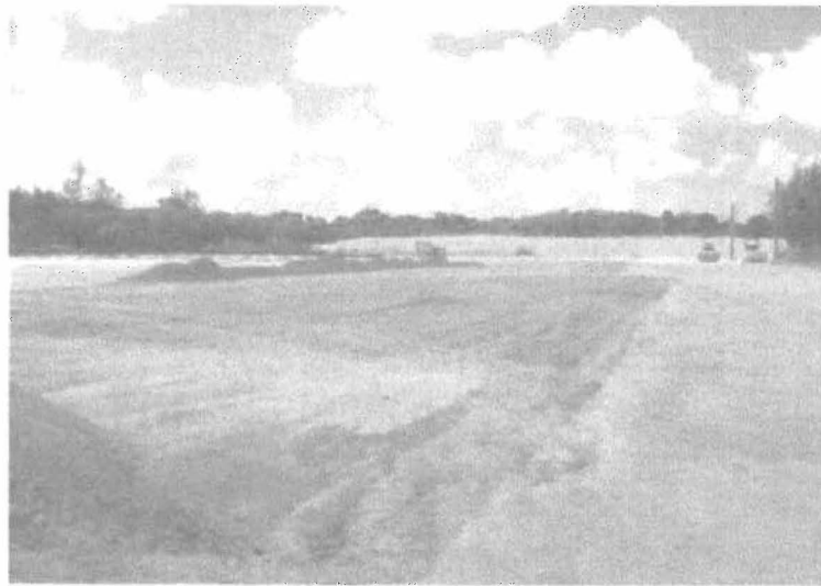
Photo 5 - Standing on existing pavement in the Basic Bid looking south
