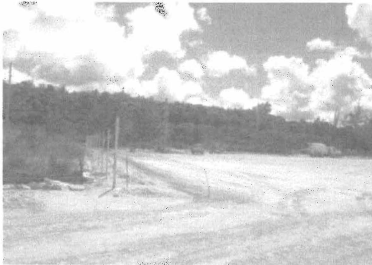
Photo 6 - Fence posts set in concrete looking east towards Marine Dr
